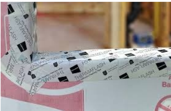
DIAGRAM 12 – bottom butterfly strip
