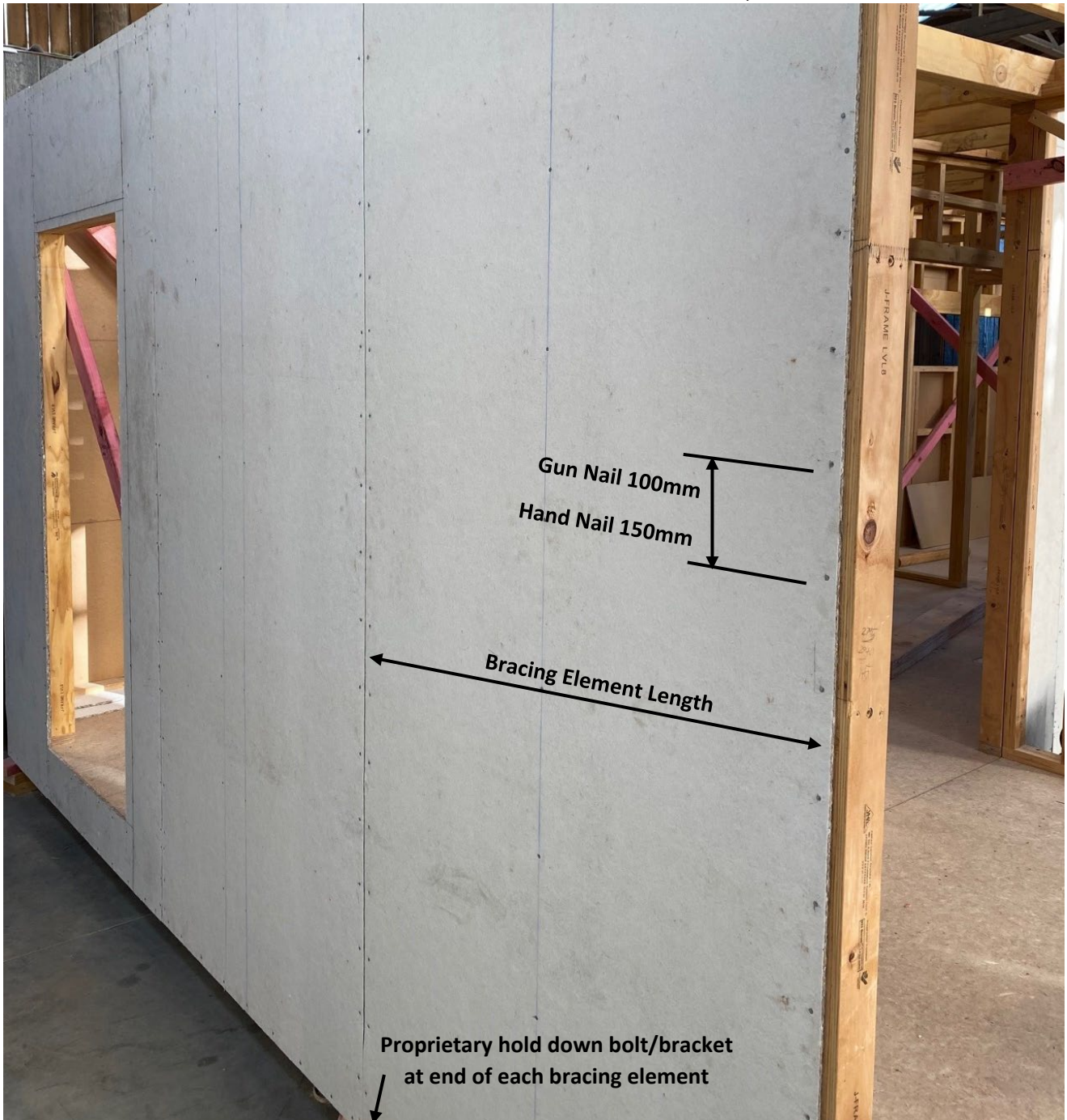
DIAGRAM 5 – Bracing Board fixings
