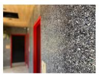
saveBOARD MultiUse used as an internal wall linings should be fixed at 600mm centres. We recommend a 2-4mm vertical gap between sheets to allow for thermal expansion during periods of high humidity (summer).
