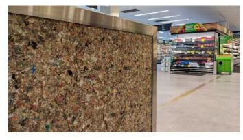
paper board and plastic waste collected in stores into saveBOARD building materials that are being trialled in stores. Subject to trial success, Woolworths will roll out saveBOARD as an integral part of its new store builds and annual refurbishment programme.
