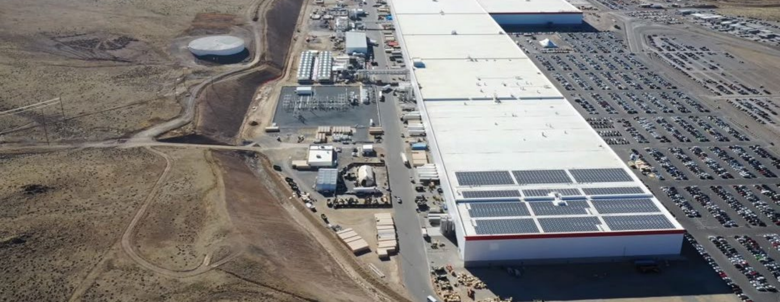
Commercial example (USA version) saveBOARD Roofing Substrate Tesla Gigafactory, Sparks Nevada, USA.
