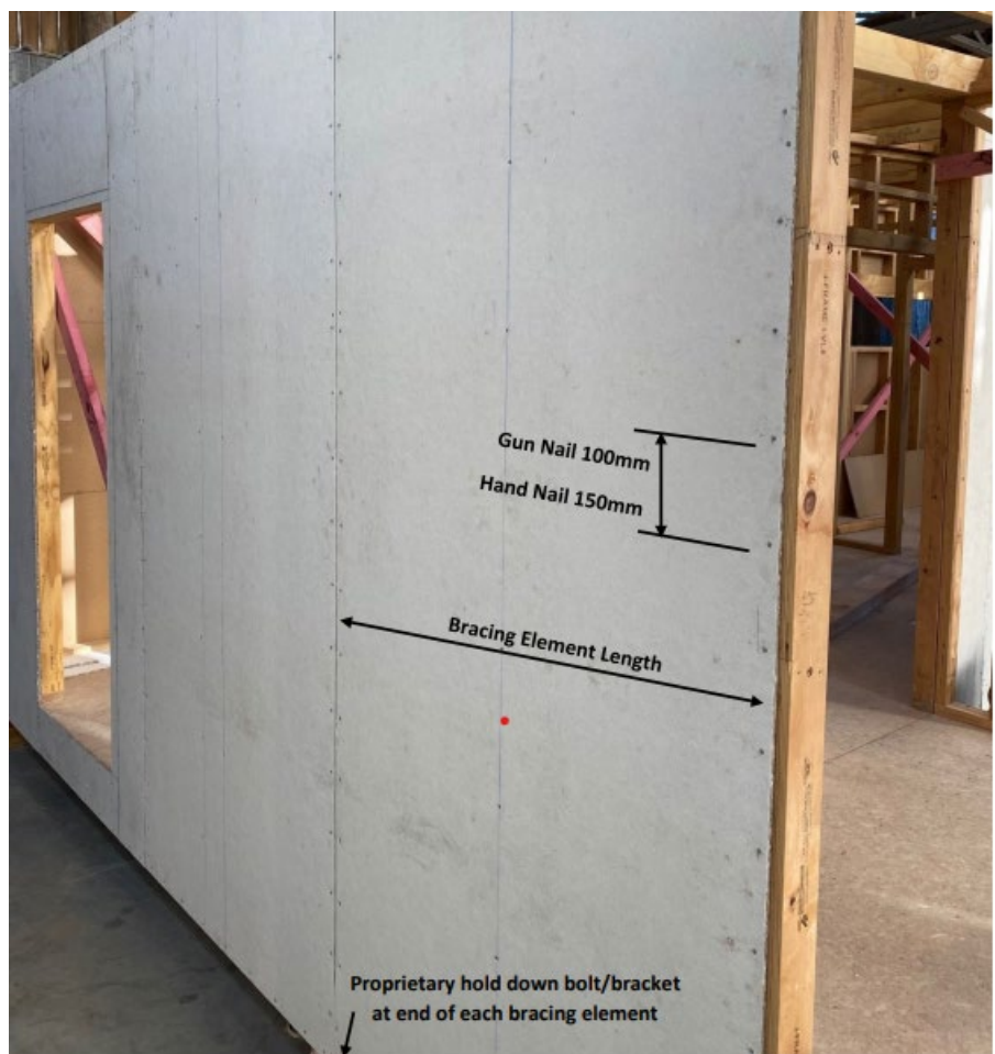
DIAGRAM 5 – Bracing Board fixings
