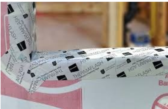
DIAGRAM 10 – bottom butterfly strip
