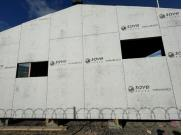
The off-cuts from the building as well as the soft plastic construction waste is being recycled back into saveBOARD, leaving no waste and creating a circular economy. Every month the use of saveBOARD will divert approximately 2,500 kg of waste from landfill.
